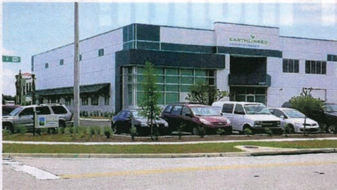
EarthLinked Technologies' Lakeland headquarters received LEED certification due in large part to use of its own technology to heat and cool the facility.
