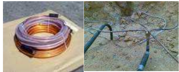
Figure 1: Copper earth loop, liquid & vapour manifold.
