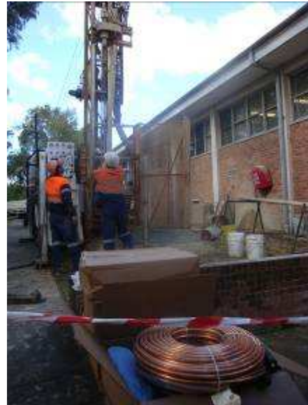
Figure 3: Installation of earth loops at CSIRO Marsfield.
