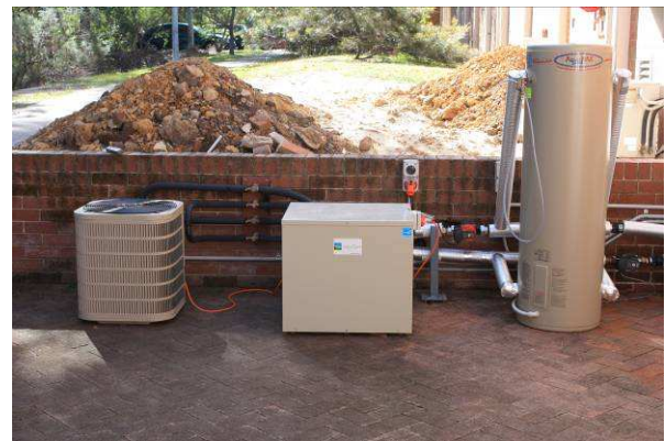
Figure 10: Location of desuperheater, compressor & buffer tank.
