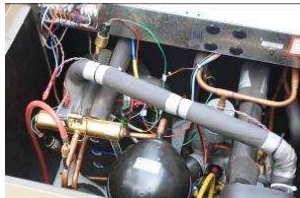
Figure 10: Location of desuperheater, compressor & buffer tank.
