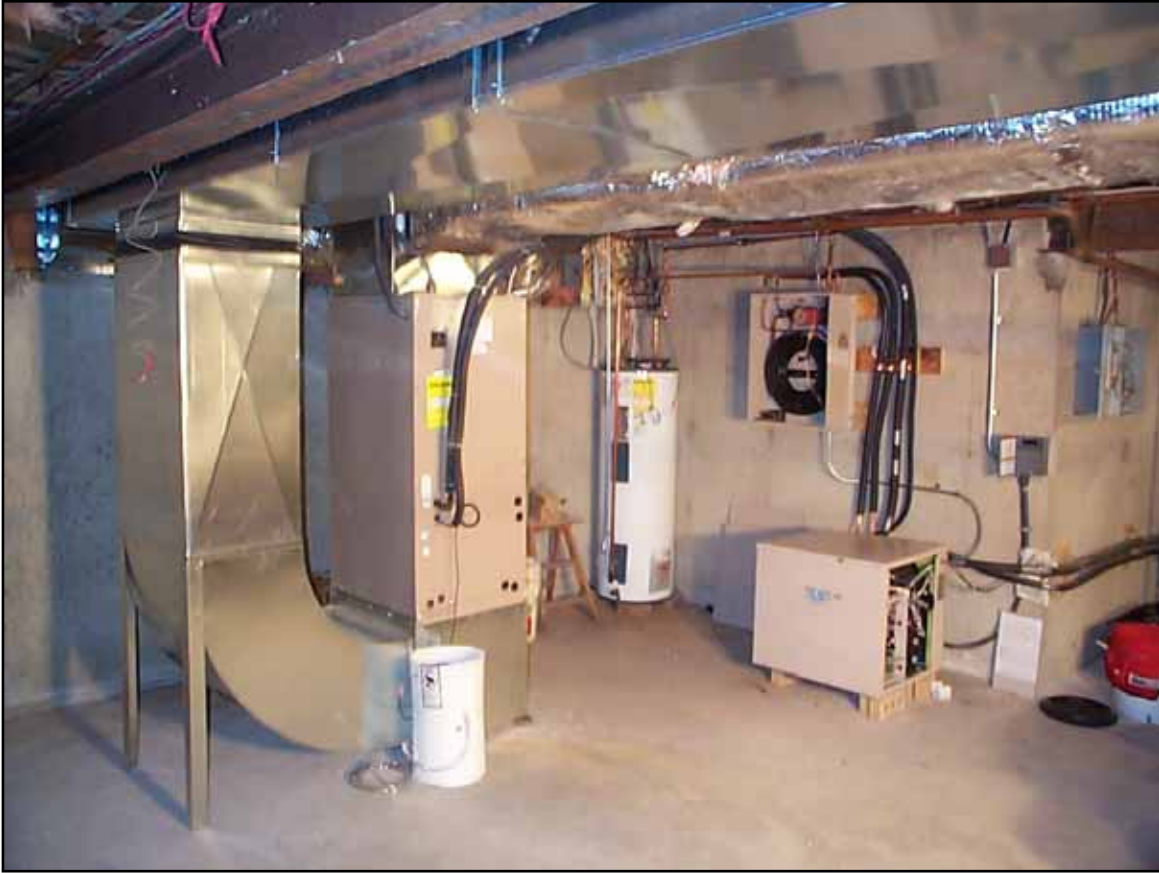
A 4-ton EarthLinked unit, air handler and heat exchanger for forced-air space heating and cooling, and domestic water heating.
