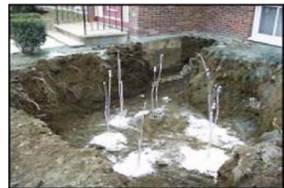
DX ground loop being installed at Claremont Arms Apartments. Six boreholes were drilled, with a copper U-loop tube in each. Tubes will be attached to supply and return headers, about 5 ft below grade, and inserted through the wall below the entry hall. White material is grout. [Photo by Mel Hensch.]
